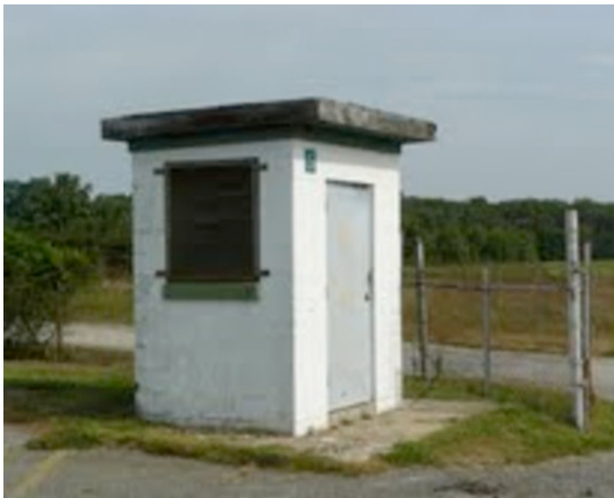
Guard house at entrance to the radar area of the Lorton NIKE missile site in Lorton. This structure was demolished in spring, 2010. Credit Irma Clifton
