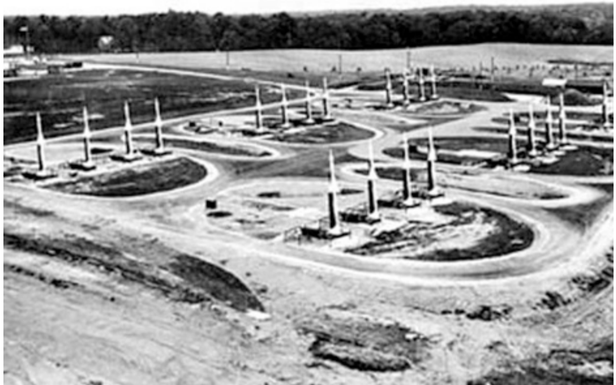
Missiles stand at alert at the Lorton NIKE missile site launch area on Furnace Road. Credit Vinton DC Public Library
