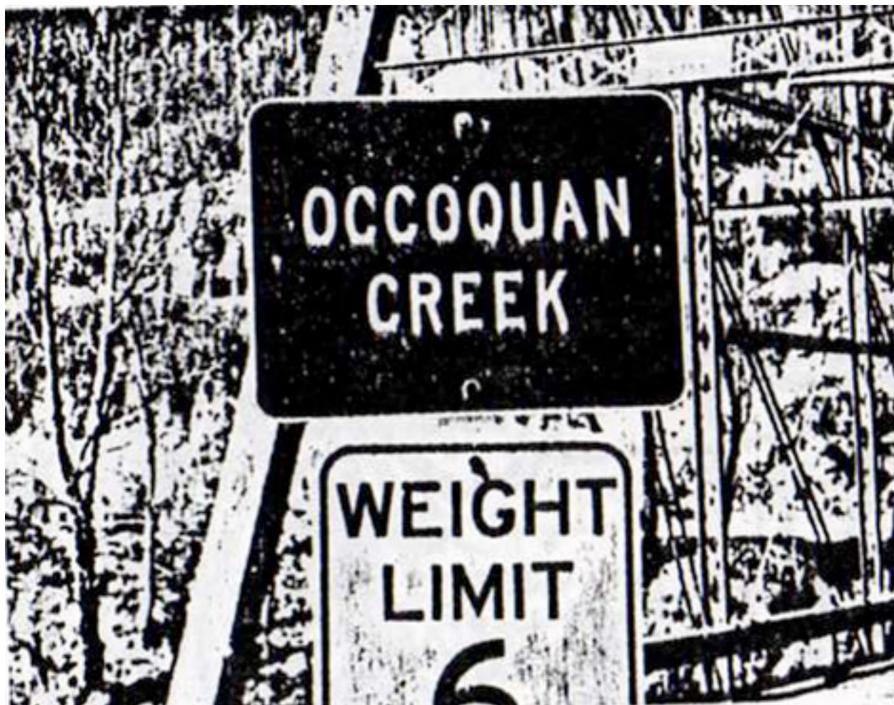
Sign affixed to the old truss bridge calling the Occoquan a creek. Credit the May 5, 1971 Potomac News.
